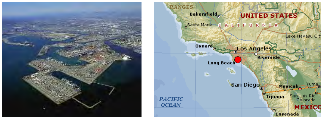
Fig. 7. Port of Long Beach, CA. The photography shows the Pier J terminal (from http://www.polb.com ). The red dot (right panel) shows the site location
