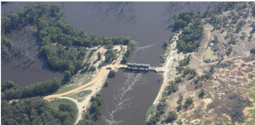
CARM will allow State Water to operate the Murrumbidgee River more efficiently and with a higher degree of precision. © DHI
