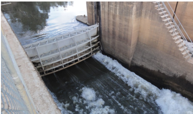
Berembed Weir diverts water into the Murrumbidgee Irrigation Area, one of the largest in Australia. © DHI
